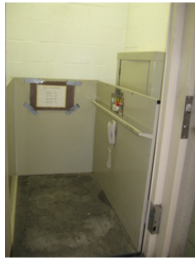
Shaft Enclosed Two-Story Lift
