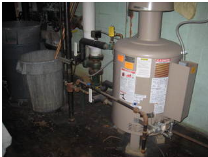
Natural Gas Fired Domestic Hot Water Heater
