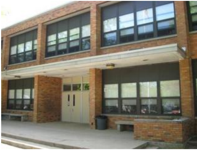
Concrete Canopy at 1953 Original Construction Main Entry
