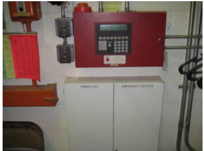
Fire Alarm System Control Panel
