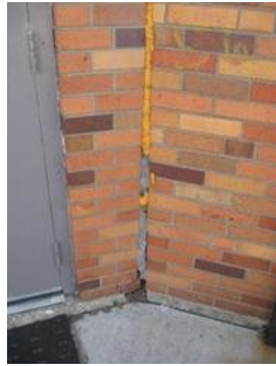
Condition of Expansion Joint in the 1953 Original Construction
