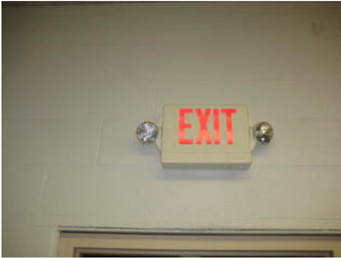
Compliant Illuminated Exit Sign
