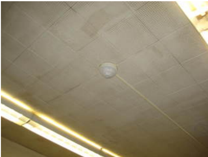
Fire Alarm System Smoke Detection Device
