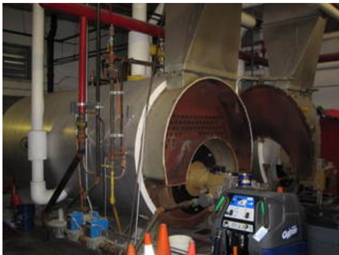
Natural Gas Fired Heated Water Boilers
