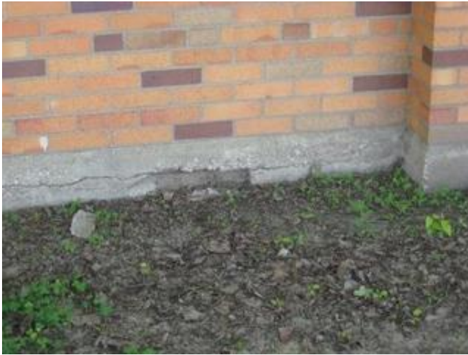
Location of Spalling in Exposed Concrete Foundation Wall
