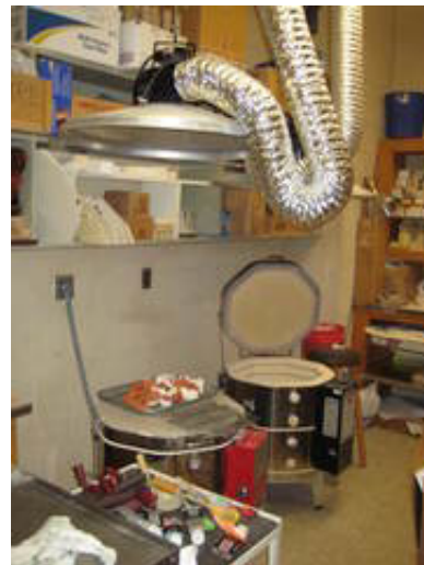
Art Program Kiln Ventilation Systems
