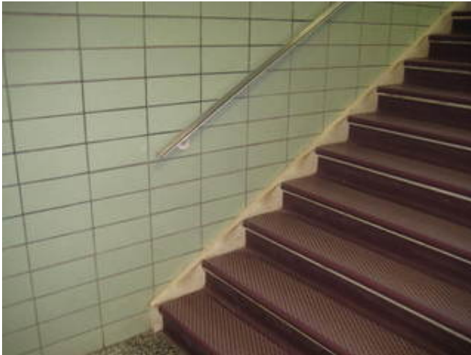
Non-Compliant Handrail
