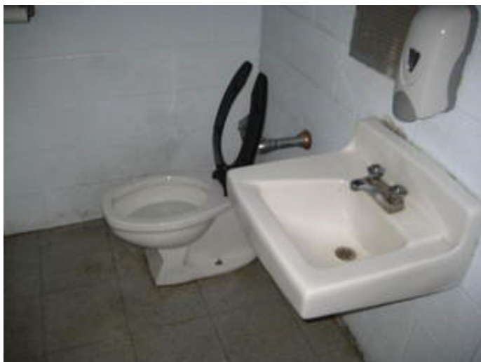
Non-ADA Floor Mounted Flush Valve Toilet and Wall Mounted Lavatory
