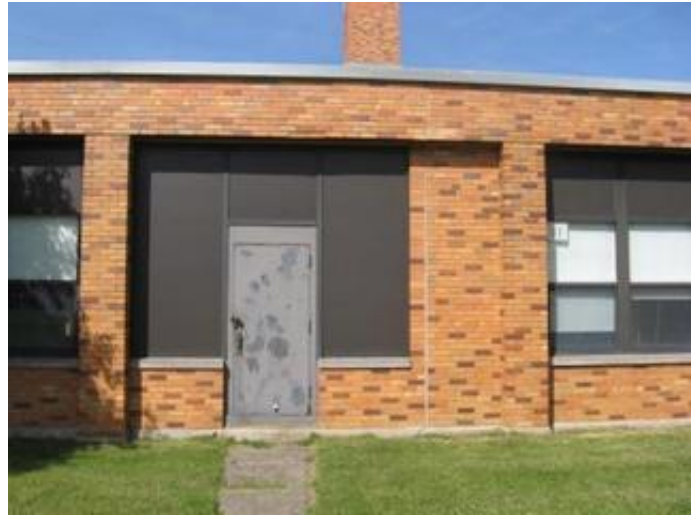
Hollow Metal Door and Frame in the 1953 Original Construction
