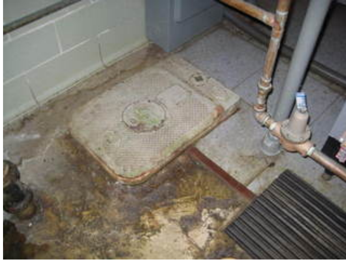
Kitchen Grease Trap Interceptor
