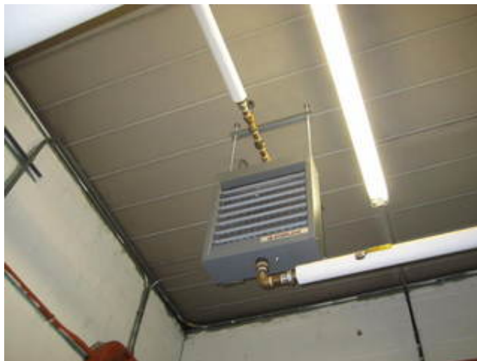
Heating Water Unit Heater
