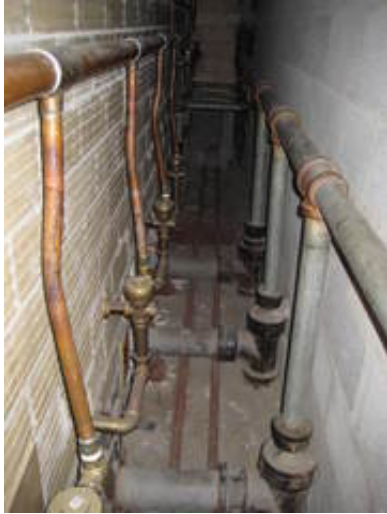
Sanitary Waste Piping
