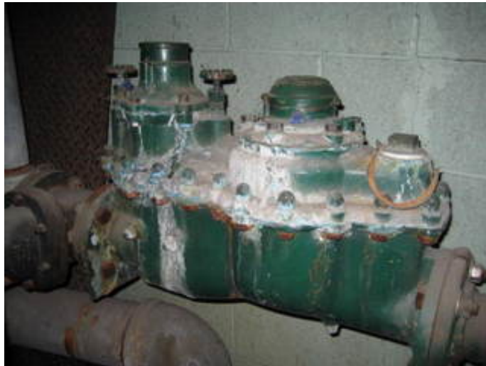
Domestic Water Supply Service Meter
