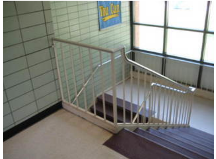
Non-Compliant Guardrail
