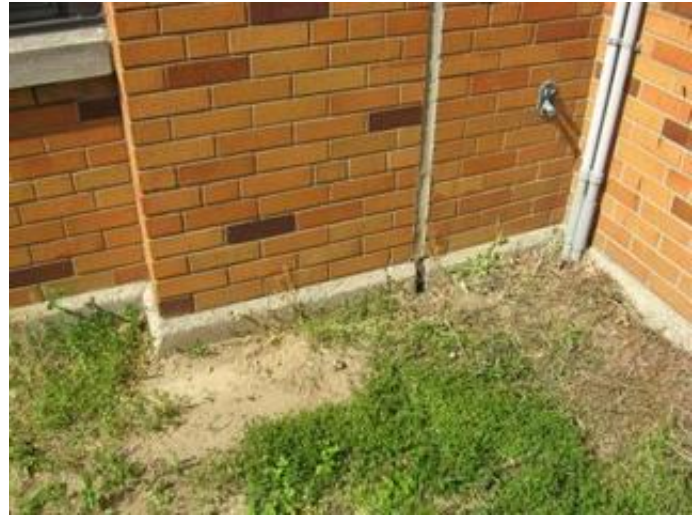
Condition of Exposed Concrete Foundation Wall at Exterior Expansion Joint
