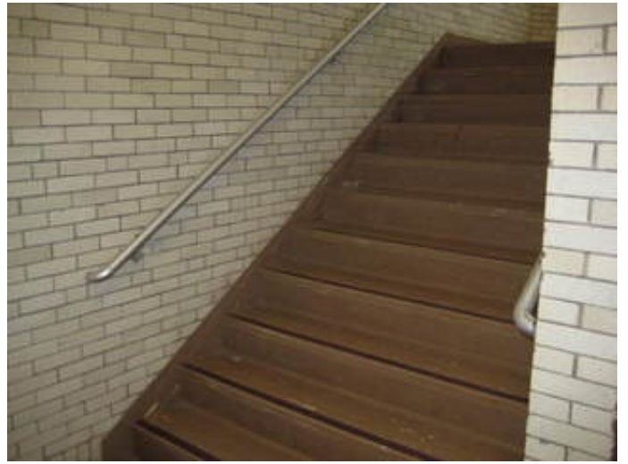
Non-compliant Handrail
