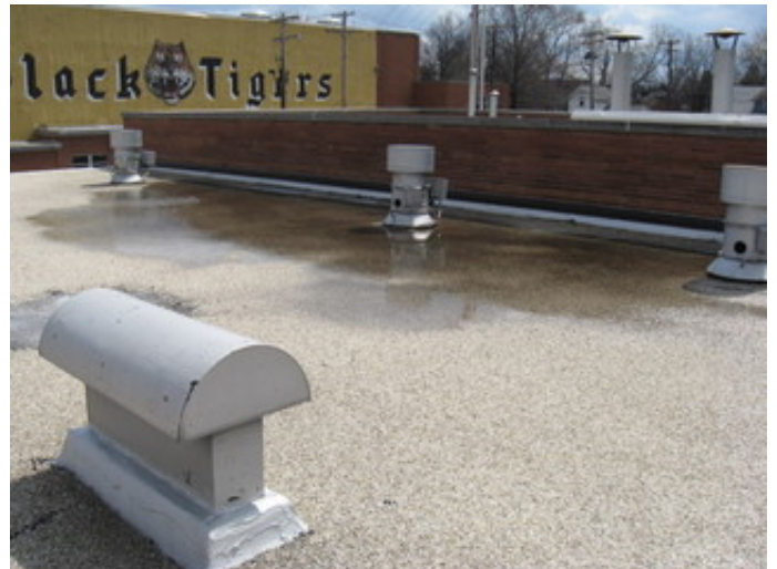
Ponding Water Over The 1927 Addition
