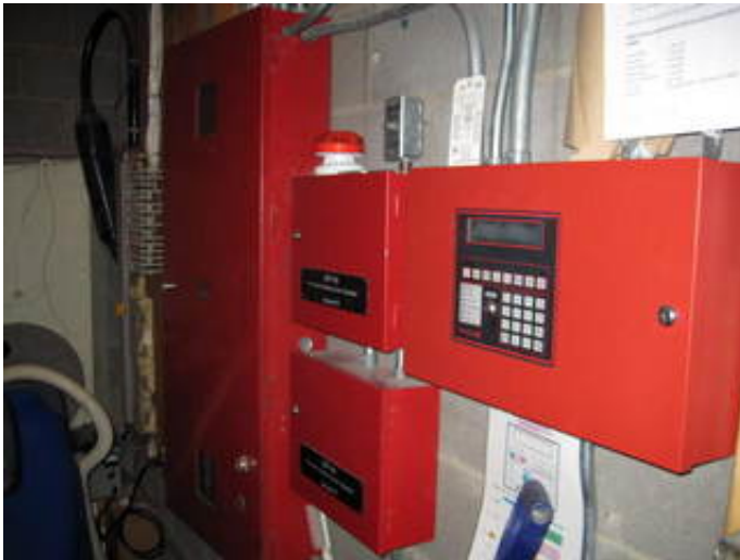
Fire Alarm, System Control Panels
