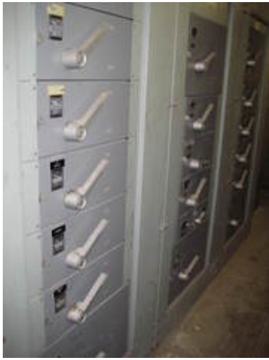
Main Electrical Distribution Panel
