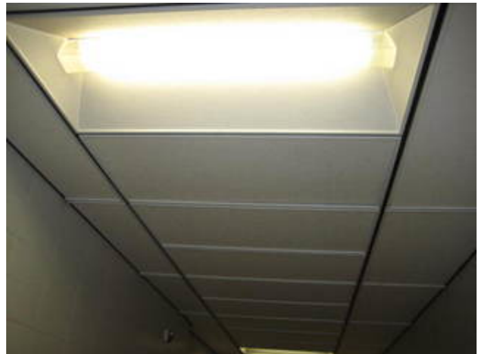
1922 Original Construction Corridor Fluorescent Light Fixture
