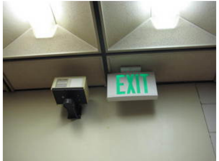
Non-compliant Green Lettered Illuminated Exit Sign
