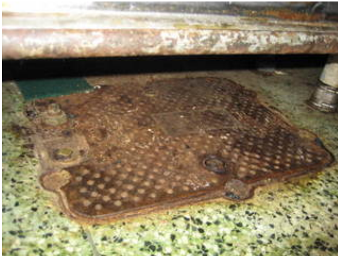
Kitchen Grease Trap Interceptor
