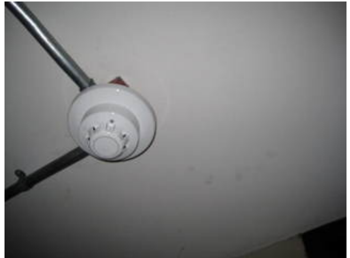
Fire Alarm System Smoke Detection Device
