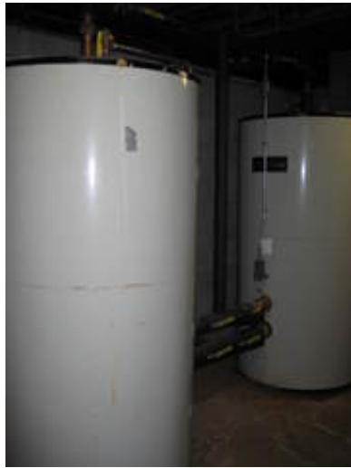
Domestic Hot Water Storage Tanks
