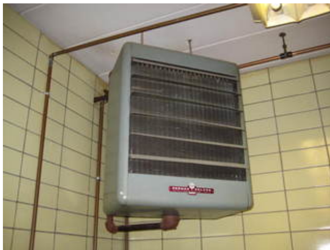
Heating Water Unit Heater
