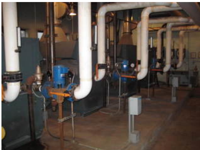
Natrual Gas Fired Heated Water Boilers
