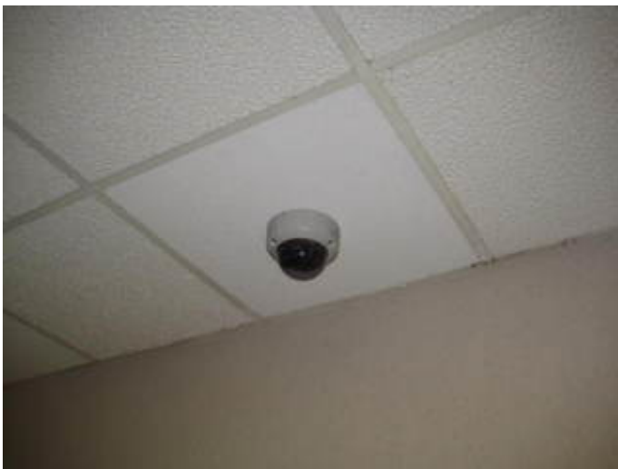
Security System CCTV Camera
