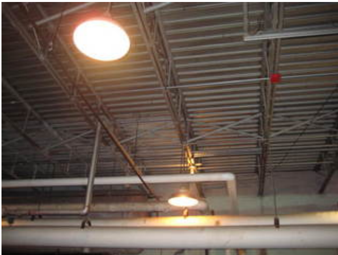
Service Area Pendant Incandescent Light Fixture
