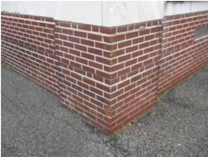
1922 Original Construction Exterior Wall at Grade
