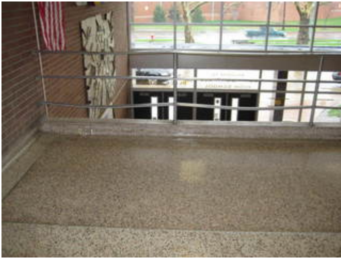
Non-compliant Guardrail
