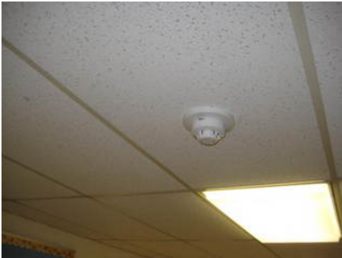
Fire Alarm System Smoke Detection Device
