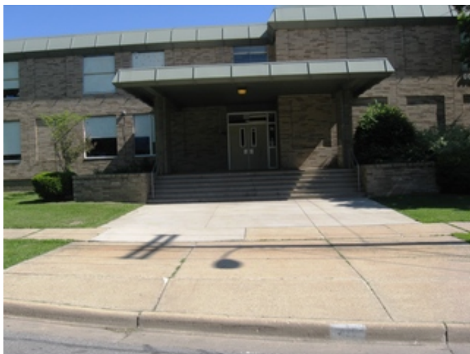
Non-Compliant ADA Access At The Main Entrance
