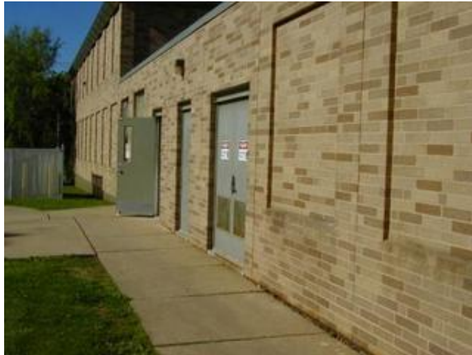
Typical Exterior Hollow Metal Doors
