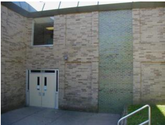
Typical Exterior Masonry Bearing Walls
