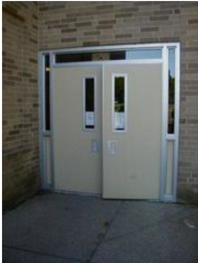
Typical Exterior FRP Entry Doors
