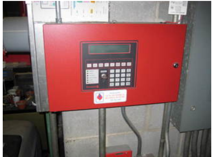
Fire Alarm System Control Panel
