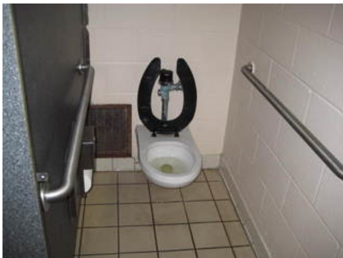
ADA Compliant Wall Hung Flush Valve Toilet
