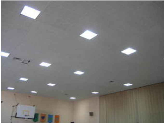
Multi-Purpose Room (Student Dining and Gymnasium) Recessed Metal Halide Light Fixtures
