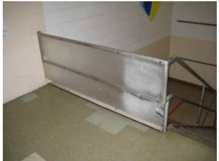
Non-Compliant Guardrail
