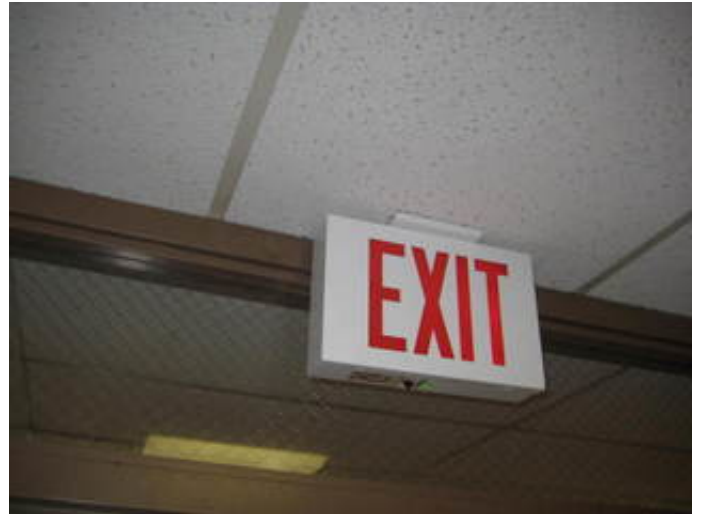
Compliant Illuminated Exit Sign
