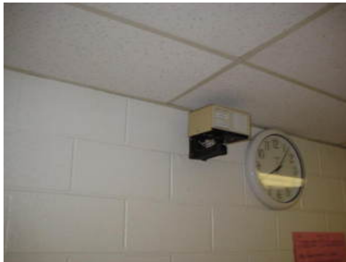
Security System Motion Detection Device
