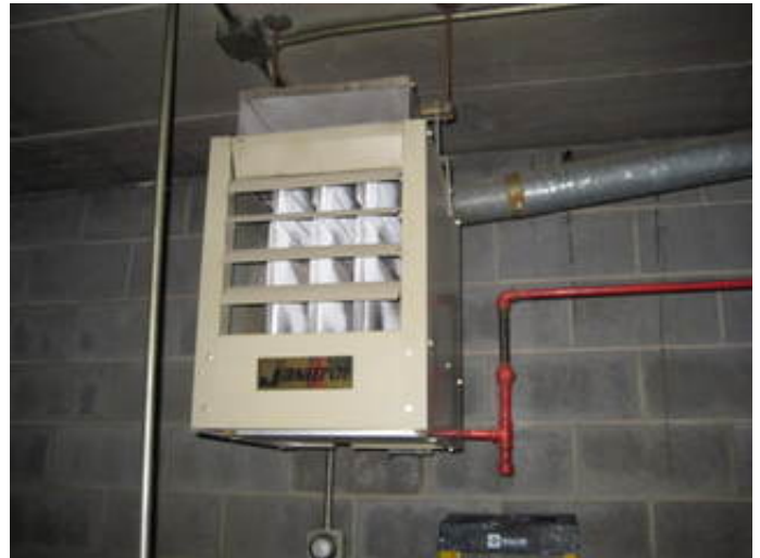
Heated Air Unit Heater
