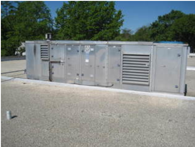
Ducted Pakaged Roof Top HVAC Unit
