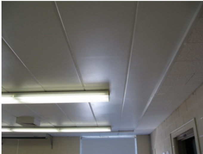
Second Floor Precast Plank Structure
