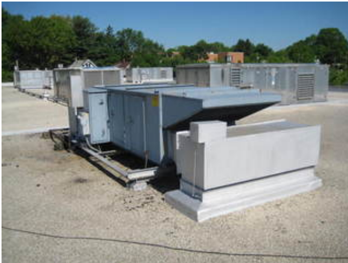
Natural Gas Fired Ducted Packaged HVAC Roof Top Unit
