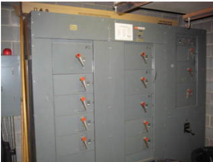
Main Electrical Distribution Panel
