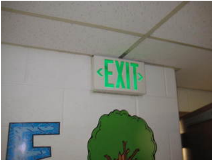
Non-Compliant Green Lettered Illuminated Exit Sign
