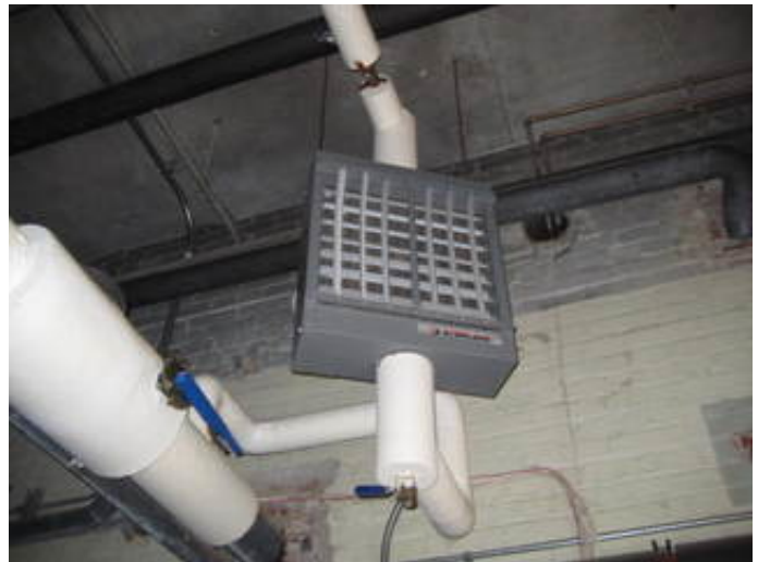
Heating Water Unit Heater
