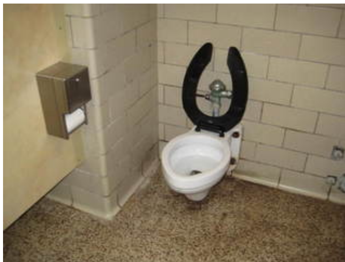
Non-ADA Wall Mounted Flush Valve Toilet
