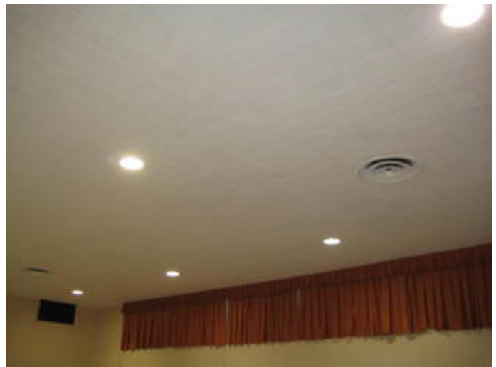
Multi-Purpose Room (Student Dining / Gymnasium) Recessed Metal Halide Light Fixtures
