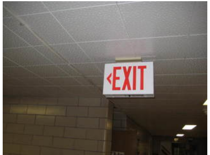
Non-Compliant Illuminated Exit Sign
