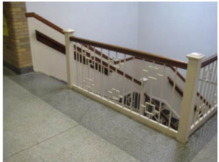
Non-Compliant Guardrail
