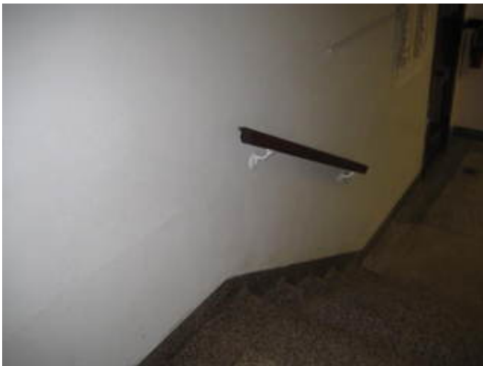
Non-Compliant Handrail
