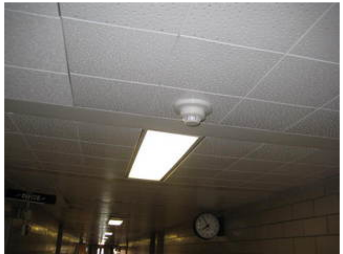
Fire Alarm System Smoke Detection Device
