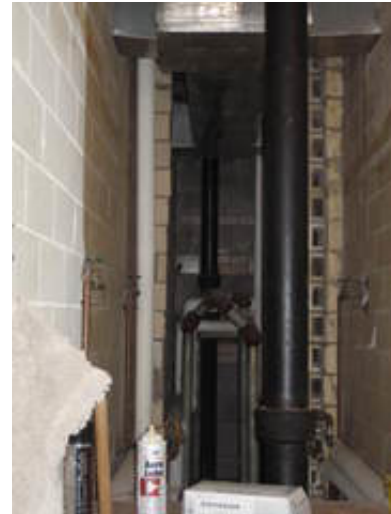
Sanitary Waste Piping
