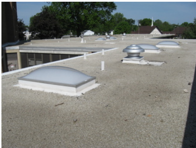
Typical Roof Over the 1959 Addition With Skylights
