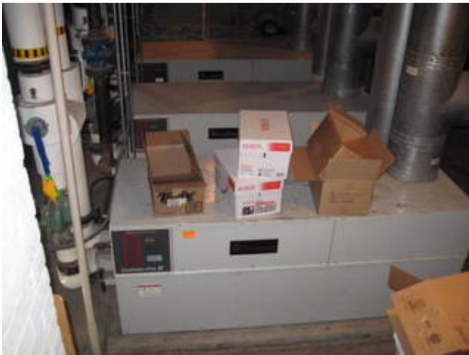
Natural Gas Fired Heated Water Boilers
