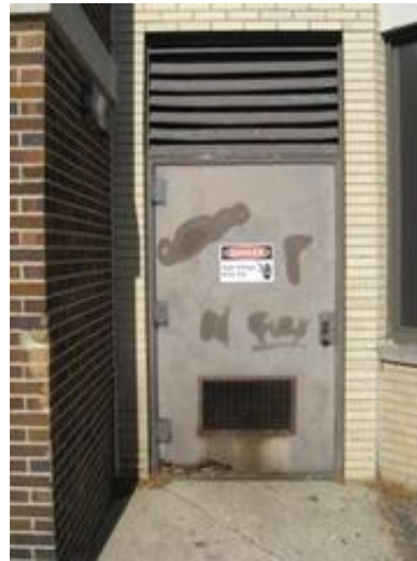
Condition of Exterior Hollow Metal Door in the 1930 Original Construction
