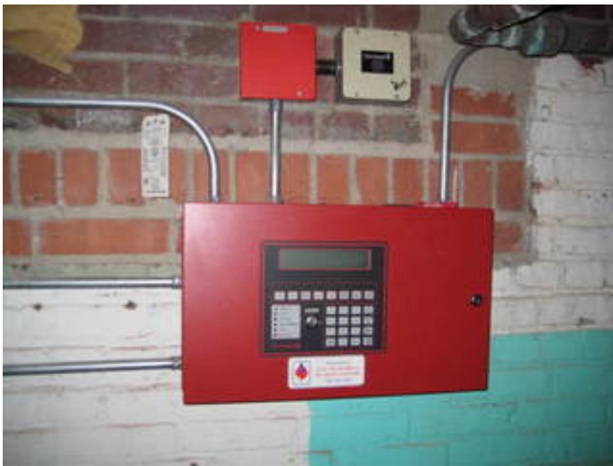
Fire Alarm System Control Panel
