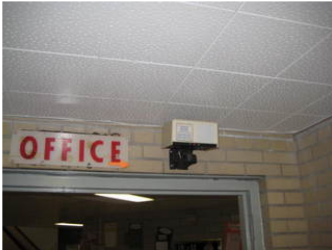
Security System Motion Detection Device
