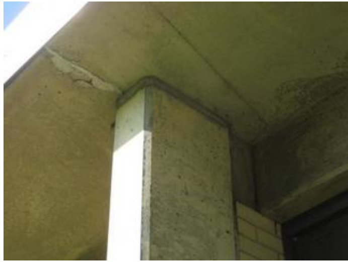
Typical Condition of Exposed Concrete Soffit and Column on the 1957 Addition
