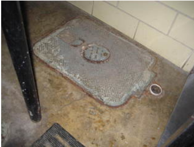
Kitchen Grease Trap Interceptor
