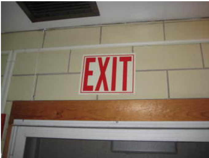
Non-Compliant Non-illuminated Exit Sign
