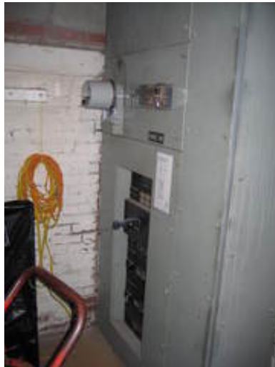
Main Electrical Distribution Panel
