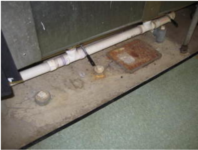
Kitchen Grease Trap Interceptor
