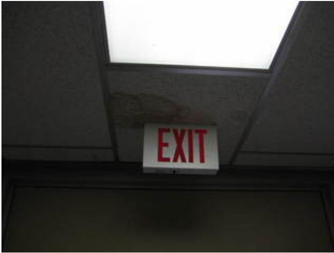
Compliant Illuminated Exit Sign
