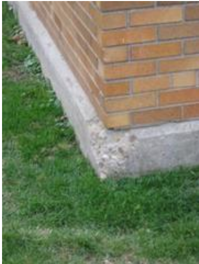
Exposed Concrete Foundation at Grade
