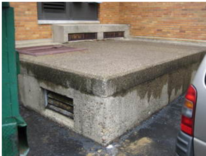
Pad Mount Transformer Vault
