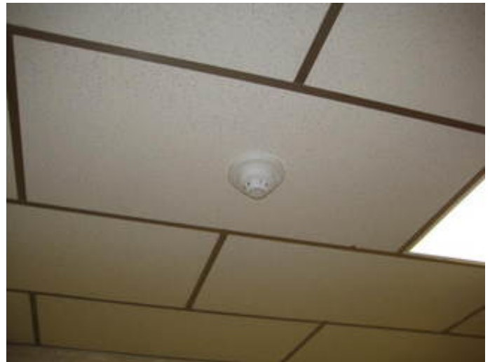
Fire Alarm System Smoke Detection Device
