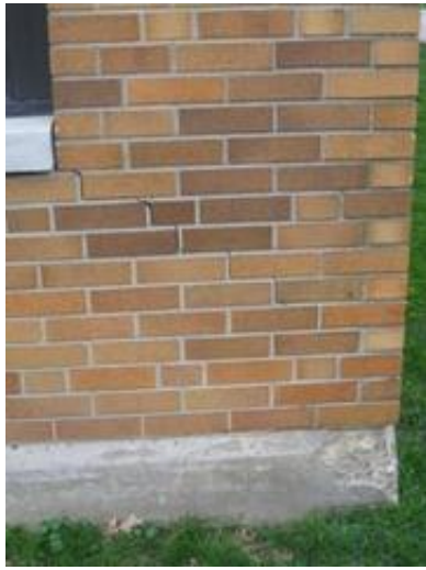
Area Requiring Masonry Repairs in the 1956 Original Construction
