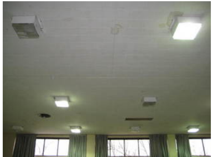
Multi-Purpose Room (Student Dining / Gymnasium) Metal Halide Light Fixtures
