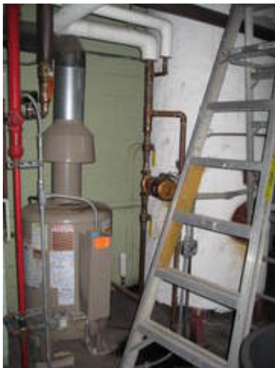
Domestic Water Heater and Storage Tank
