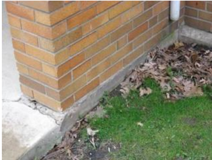
Exposed Concrete Foundation at Building Entry
