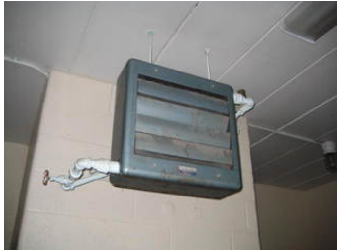
Heating Water Unit Heater
