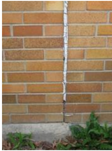
Typical Condition of Expansion Joints in Exterior Walls
