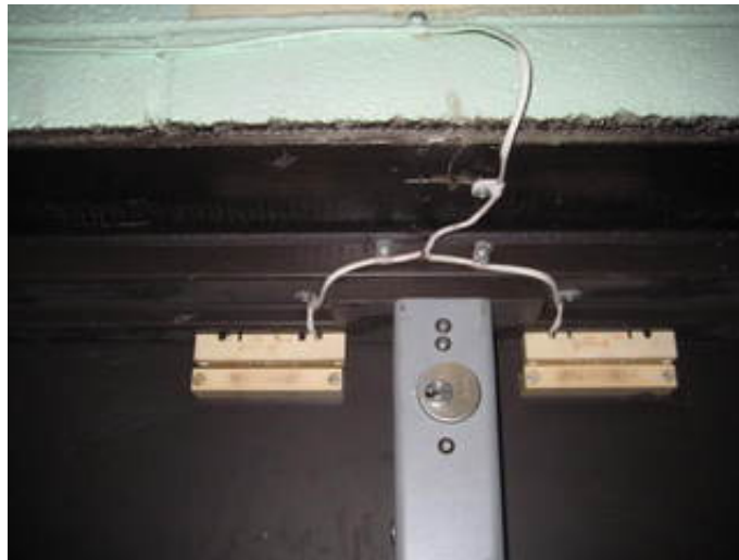
Security System Door Contact
