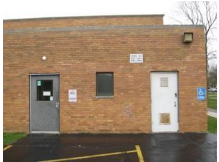
Exterior Hollow Metal Doors
