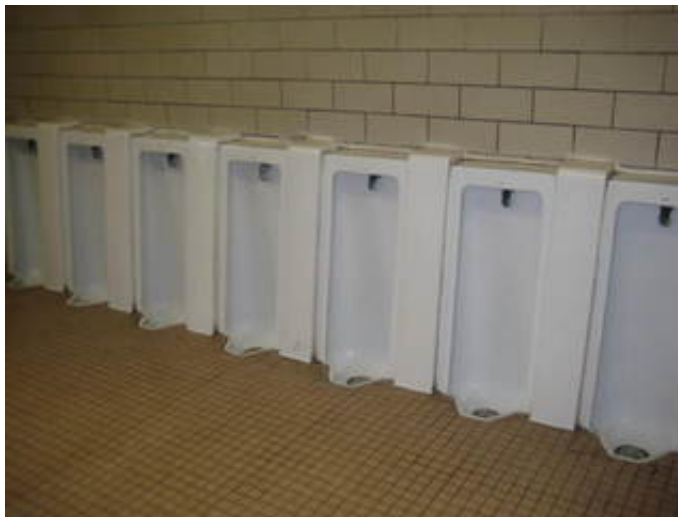
Central Flush Floor Mounted Urinals
