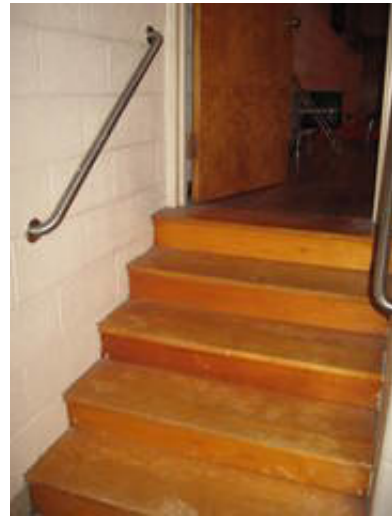
Non-Compliant Handrails At the Stage Steps
