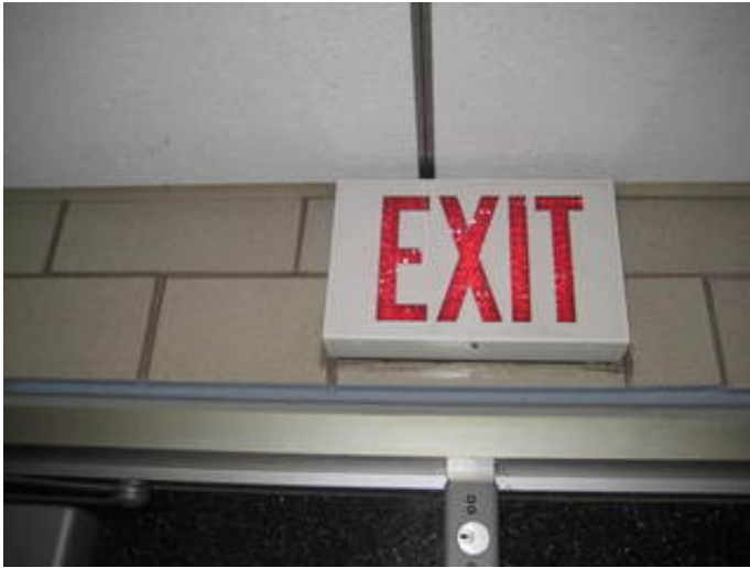
Compliant Illuminated Exit Sign
