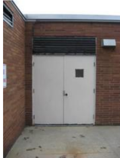
Exterior Hollow Metal Doors in the 1958 Original Construction
