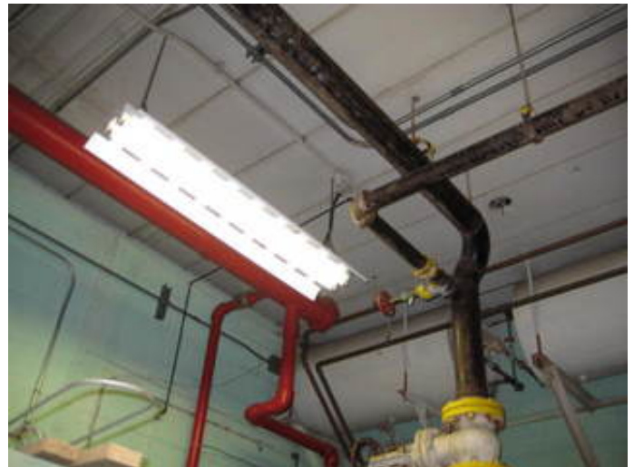
Service Area Suspended Fluorescent Light Fixture
