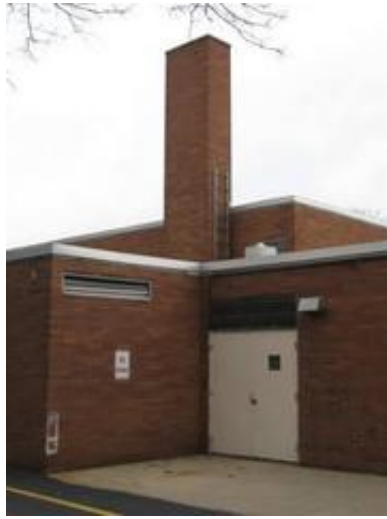
Exterior Masonry and Chimney in the 1958 Original Construction
