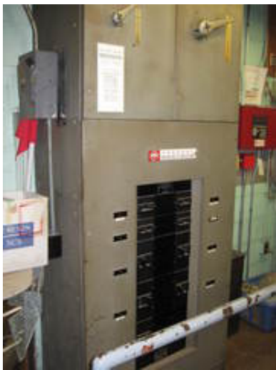
Main Electrical Distribution Panel
