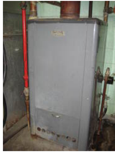
Domestic Hot Water Boiler
