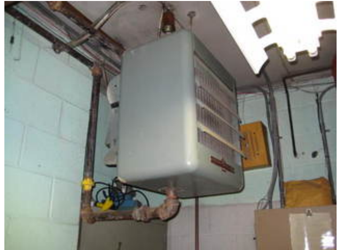
Heating Water Unit Heater
