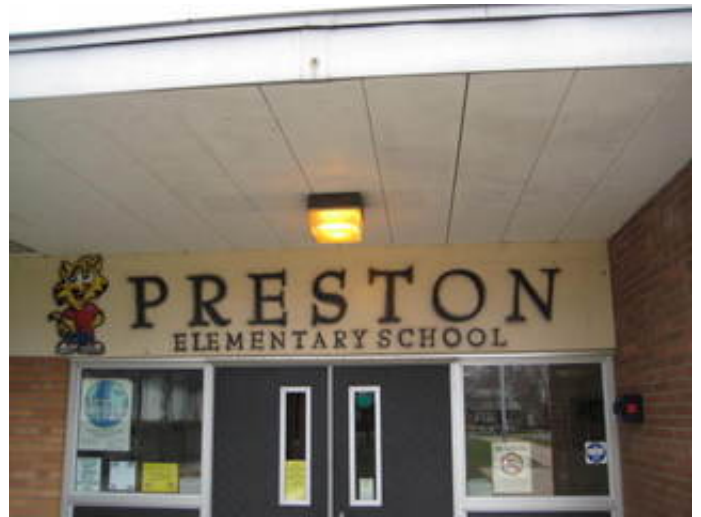
Surface Mounted HID High Pressure Sodium Entry Light Fixture
