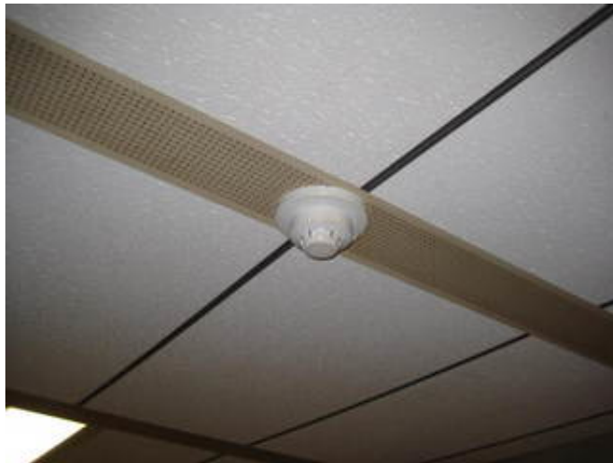
Fire Alarm System Smoke Detection Device
