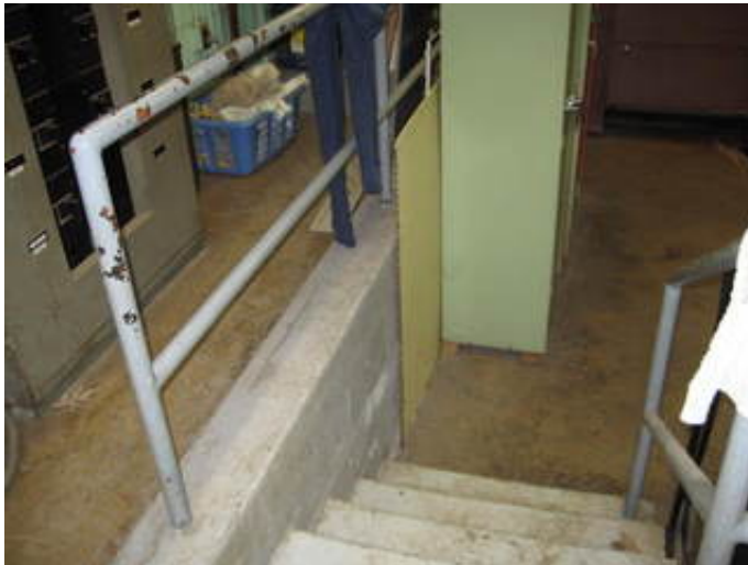
Mechanical Room Non-compliant Guardrail and Handrail
