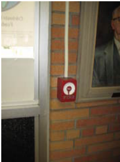
Fire Alarm System Manual Pull Station
