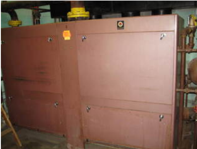
Natural Gas Fired Heated Water Boilers
