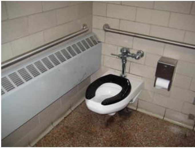
ADA Compliant Wall Hung Flush Valve Toilet
