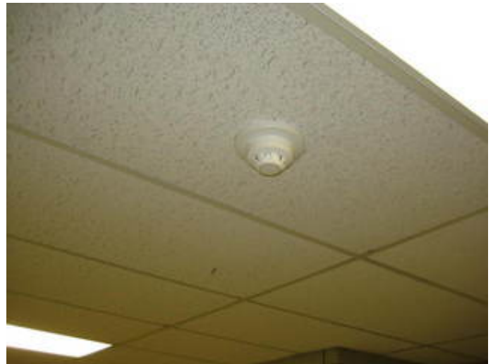
Fire Alarm System Smoke Detection Device
