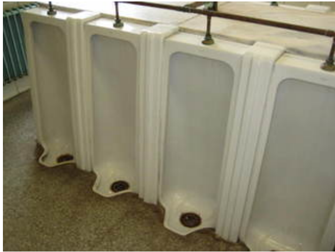
Central Flush Floor Mounted Urinals
