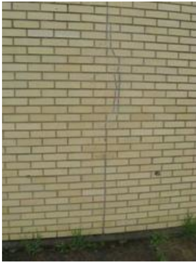
Area of Exterior Masonry Wall Requiring Repairs
