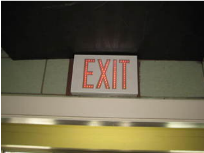
Compliant Illuminated Exit Sign
