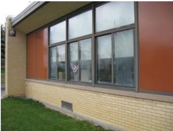
Typical Classroom Windows with Broken Glazing Seals
