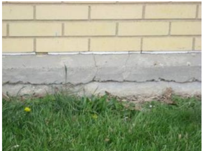
Typical Condition of Exposed Concrete Foundation Wall at Grade
