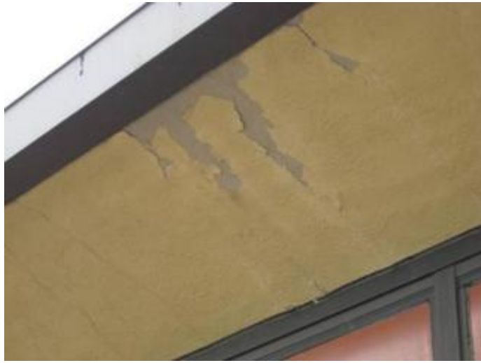
Typical Condition of Exterior Plaster Soffit Over Classroom Windows
