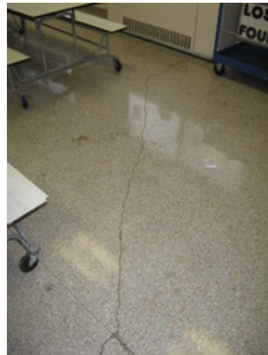
Crack In Floor Slab-On-Grade of Student Dining
