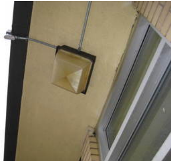
Surface Mounted HID High Pressure Sodium Light Fixture
