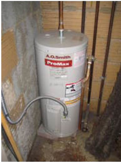
Electric Domestic Water Heater
