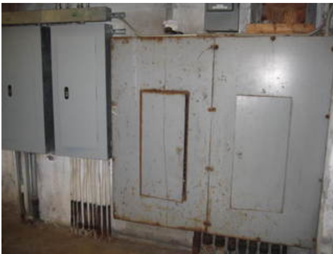
Main Electrical Distribution Panel
