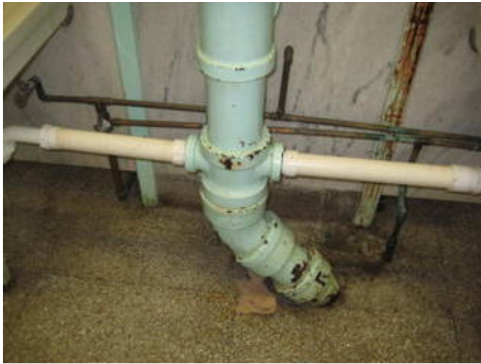
Sanitary Waste Piping
