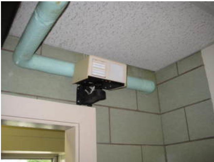
Security System Motion Detection Device
