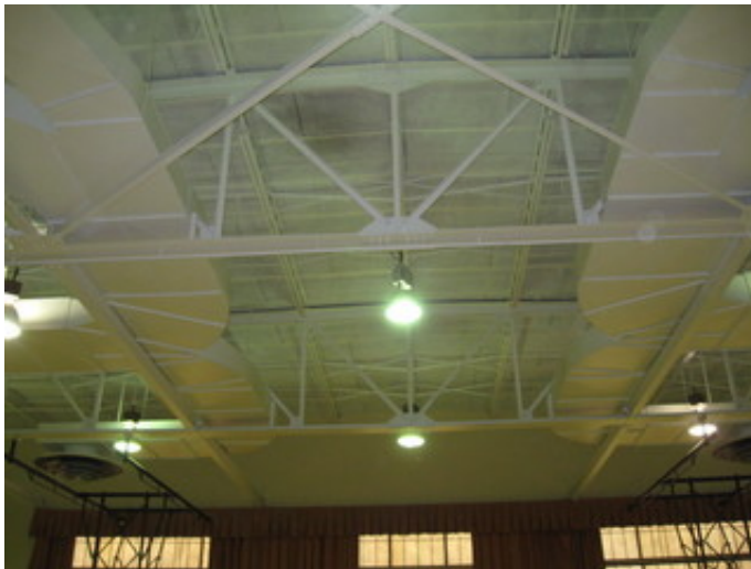
Typical Roof Structure Over the Gymnasium
