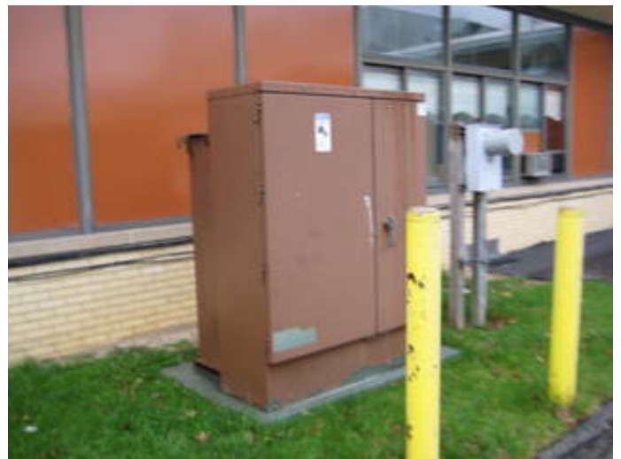
Pad Mounted Transformer
