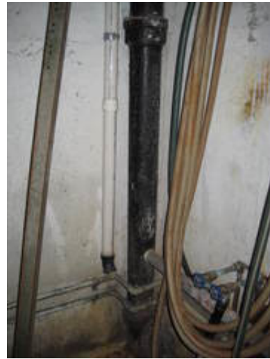
Sanitary Waste Piping
