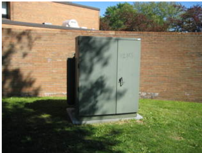
Pad Mounted Transformer
