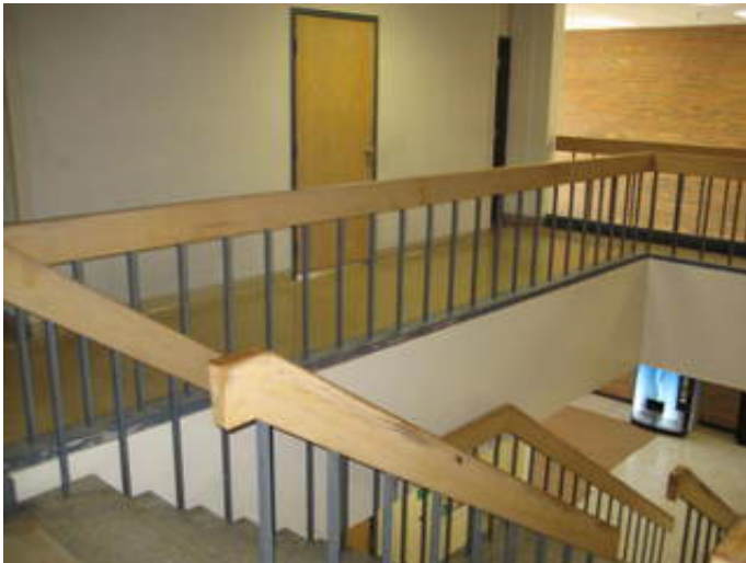
Non-Compliant Guardrail
