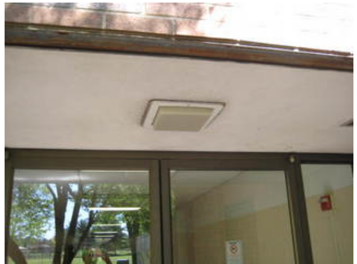
Recessed HID High Pressure Sodium Entry Light Fixture
