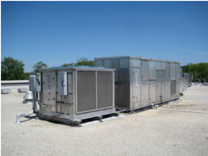
Ducted Packaged Roof Top HVAC Unit
