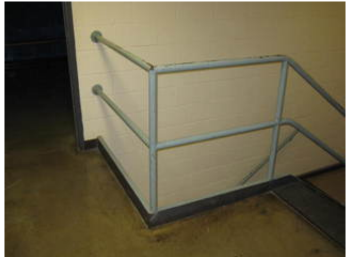
Non-Compliant Guardrail
