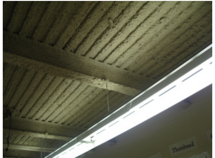
Floor Construction Of The Second Floor
