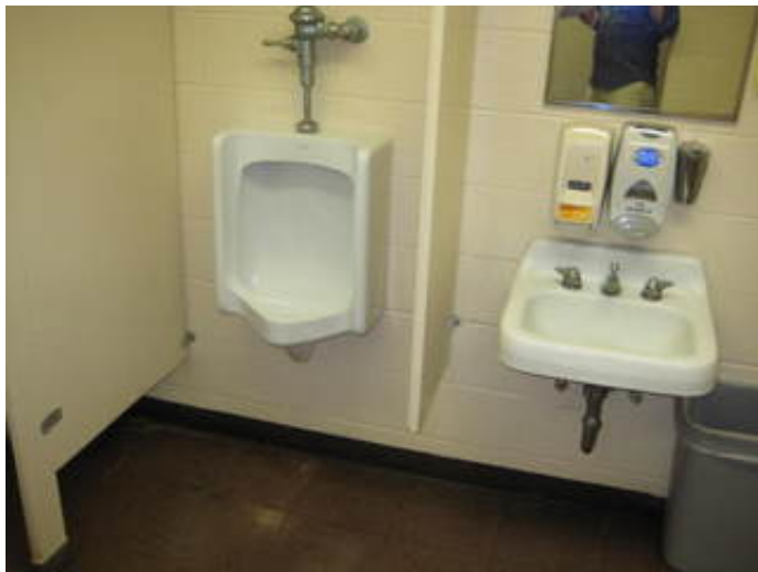
Non-ADA Wall Hung Flush Valve Urinal and Wall Hung Lavatory
