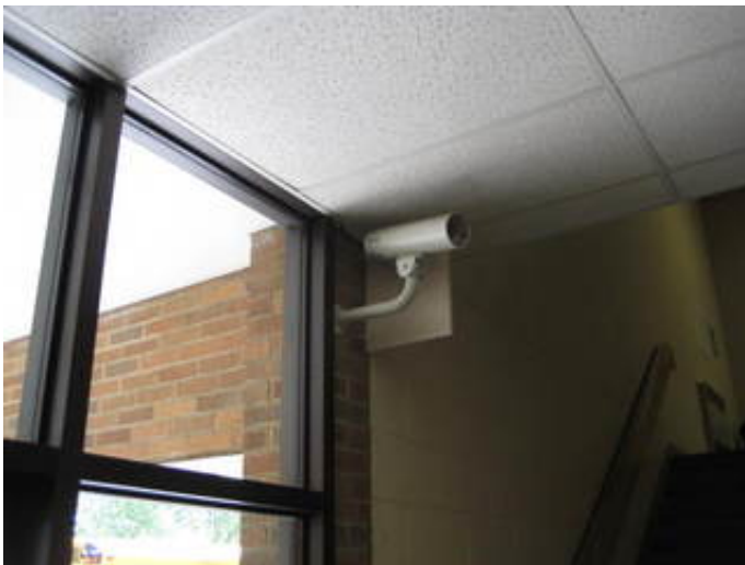
Security System CCTV Camera
