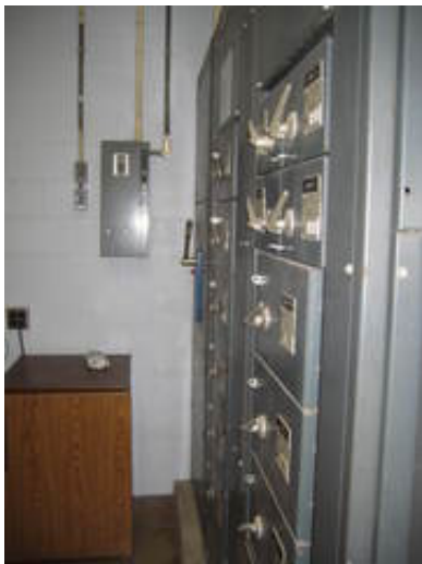
Main Electrical Distribution Panel
