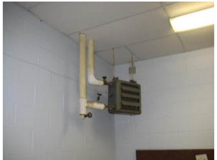
Heating Water Unit Heater
