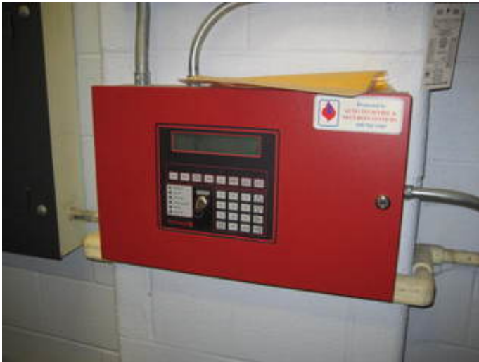
Fire Alarm System Control Panel
