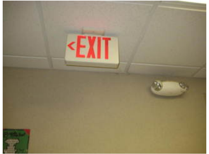
Compliant Illuminated Exit Sign
