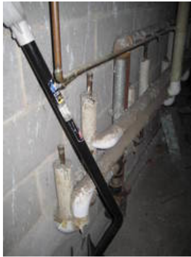
Sanitary Waste Piping
