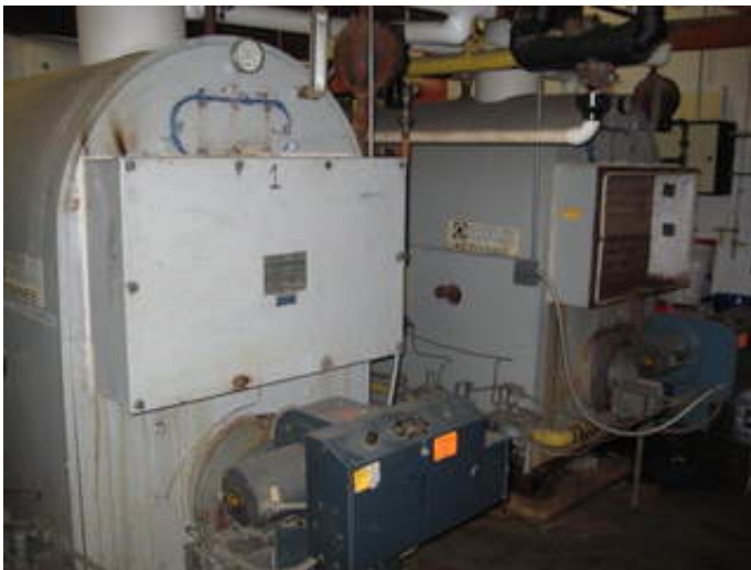
Natural Gas Fired Heated Water Boilers
