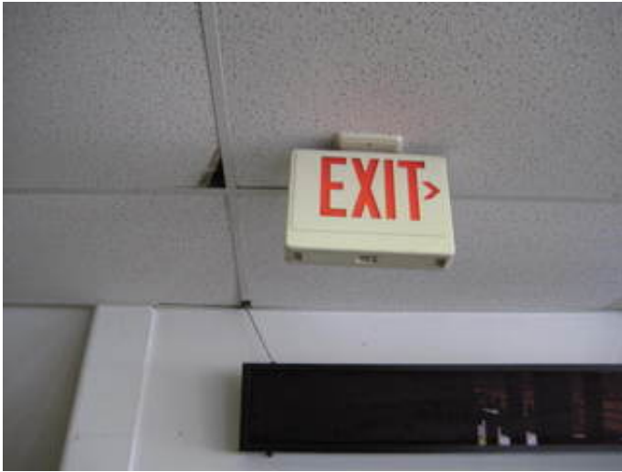
Non-Compliant Plastic Construction Illuminated Exit Sign
