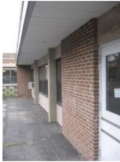
Typical Exterior Wall and Soffit
