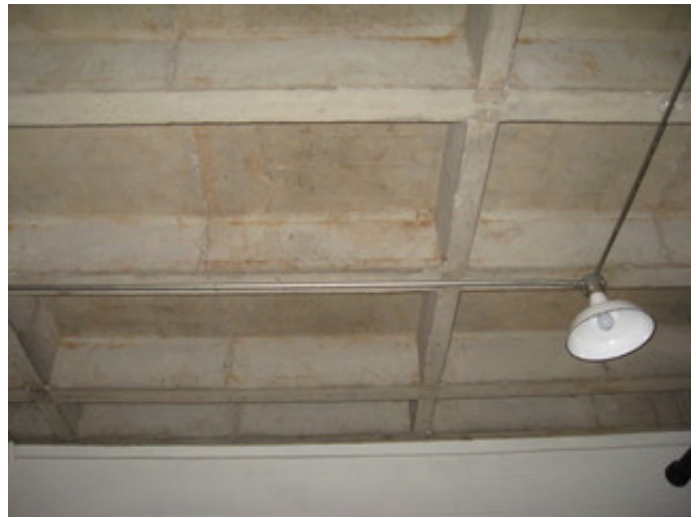
Reinforced Cast-In-Place Two-Way Concrete Slab Floor Of Elevated Classroom Wing
