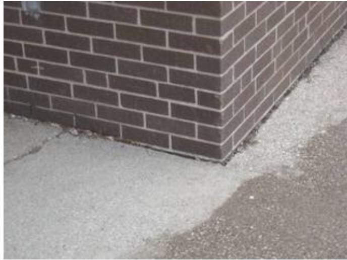
Condition of Exterior Wall Adjacent to Pavement
