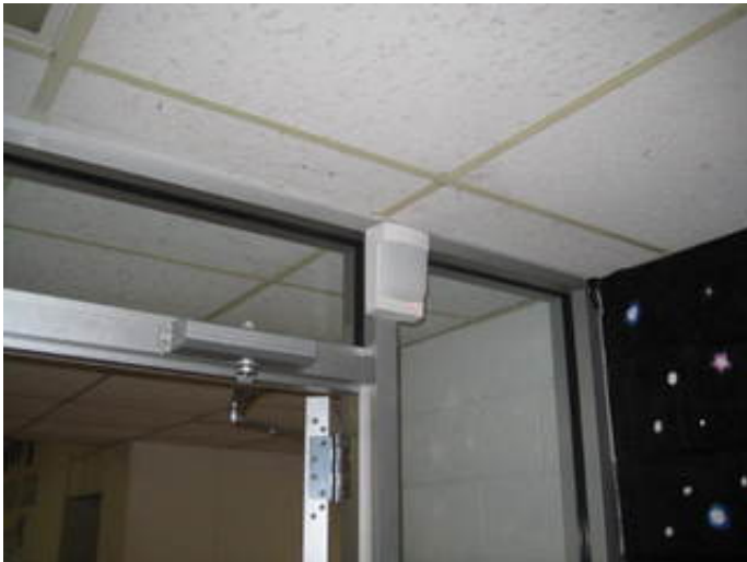
Security System Motion Detection Device
