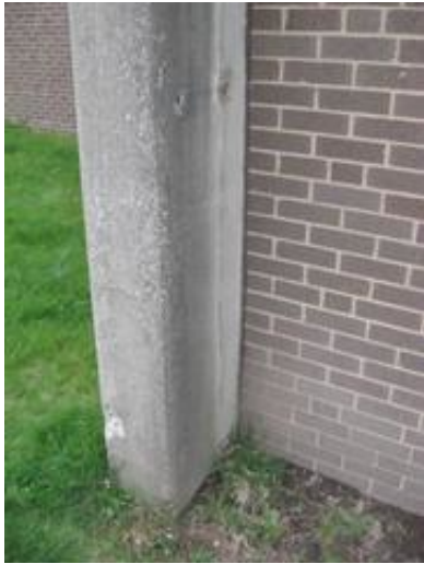
Condition of Exterior Wall and Concrete Column at Grade
