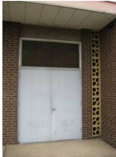
Typical Exterior Hollow Metal Doors
