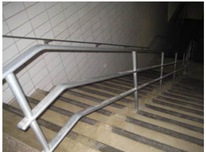
Non-Compliant Handrails
