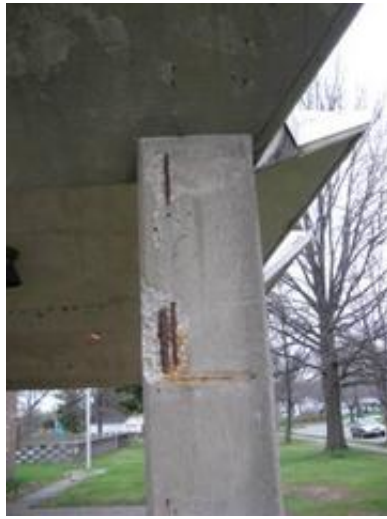
Concrete Column Support for Entry Canopy
