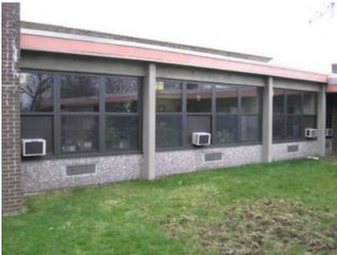
Typical Classroom Windows
