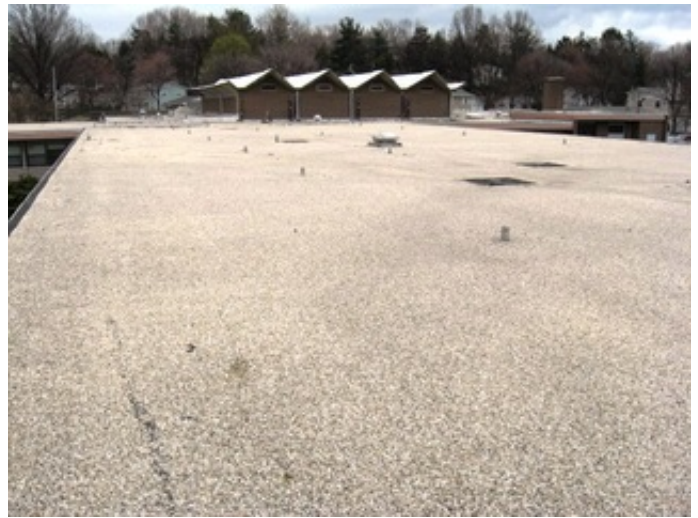
Roof Over The West Classroom Wing
