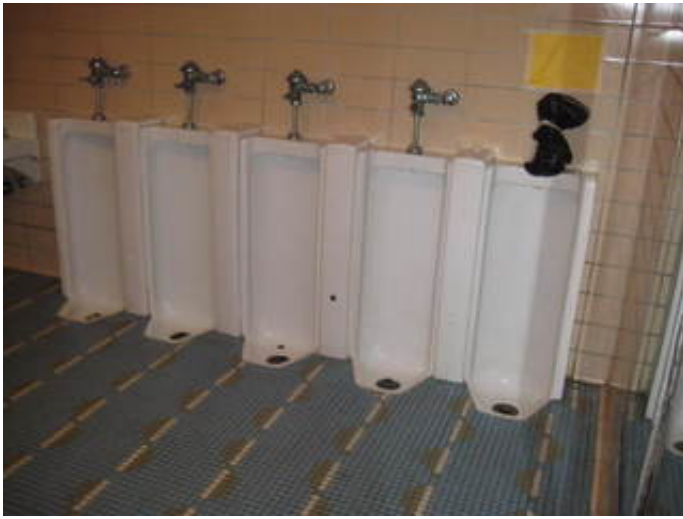
Floor Mounted Flush Valve Urinals
