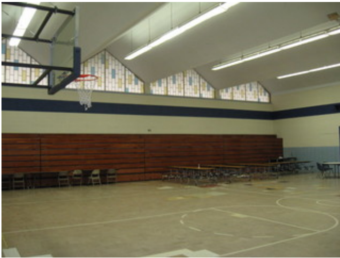
Folded Plate Concrete Roof Structure Over the Multi-Purpose Space
