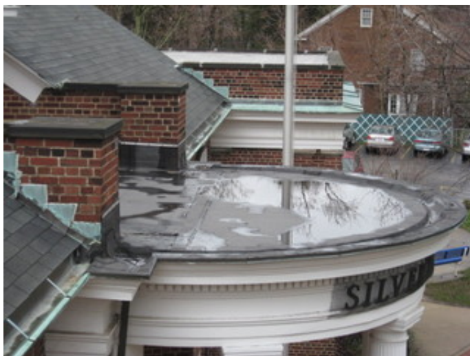
Asphalt Shingle and EPDM Roof Over the 1927 Original Construction
