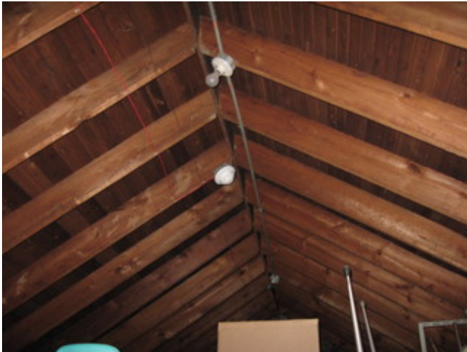
Wood Roof Structure Over the 1927 Original Construction
