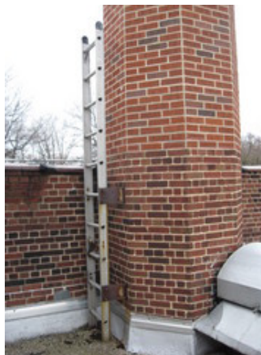
Non-Compliant Roof Ladder At the 1946 Addition
