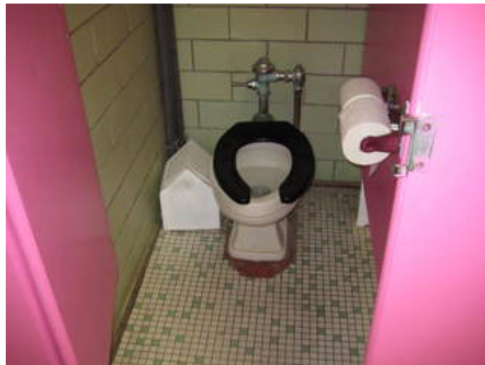
Floor Mounted Flush Valve Toilet
