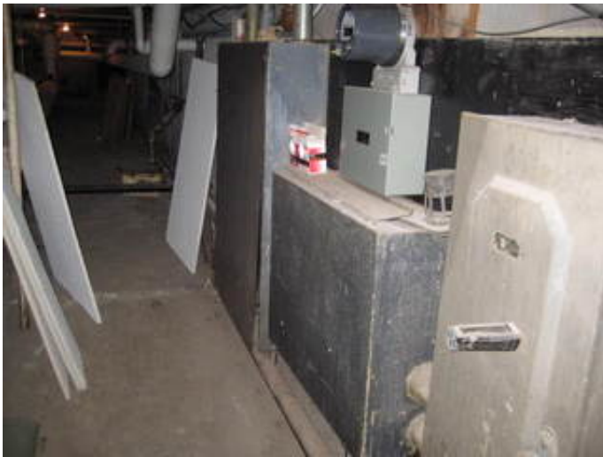
Main Electrical Distribution Panel
