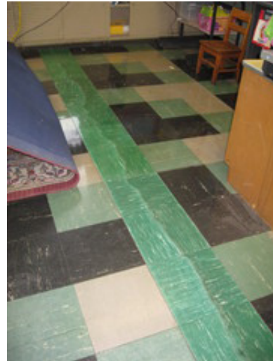
Crack In the Floor Slab In the Southwest Classroom Of the 1946 Addition
