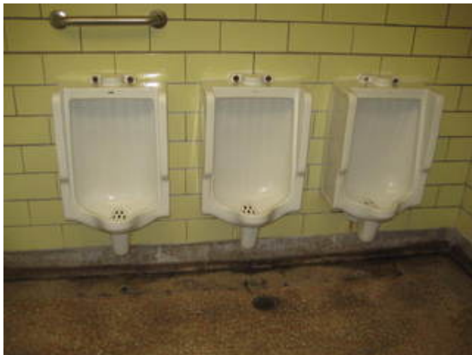
Wall Hung Central Flush Urinals
