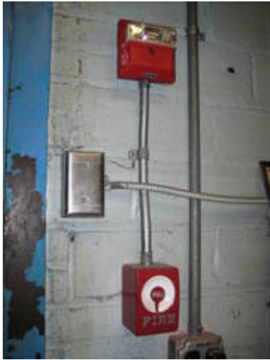
Fire Alarm System Manual Pull Station and Horn and Strobe Indication Device
