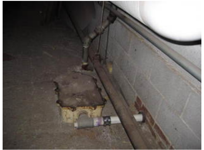
Kitchen Grease Trap Interceptor
