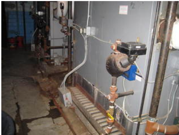
Natural Gas Fired Steam Boilers
