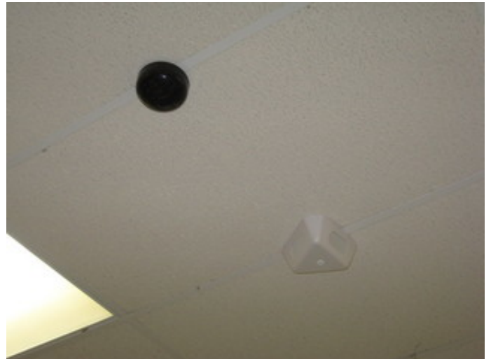
Infrared Classroom Amplification Technology System
