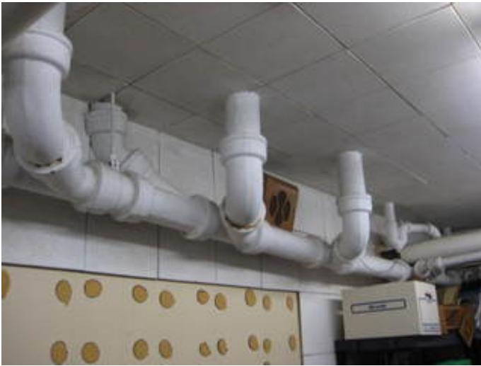
Sanitary Waste Piping
