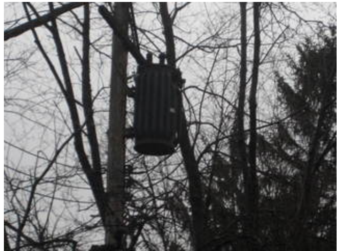
Pole Mounted Transformer
