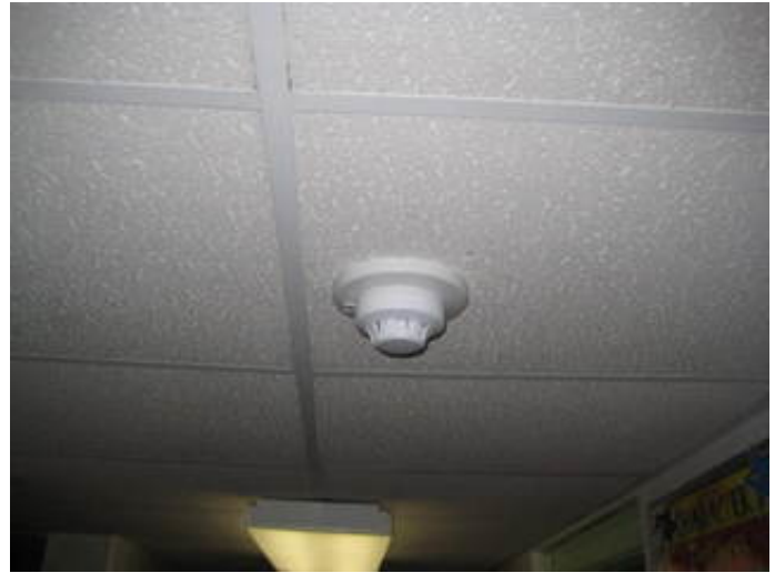
Fire Alarm System Smoke Detection Device
