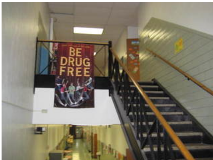
Non-compliant Guardrails
